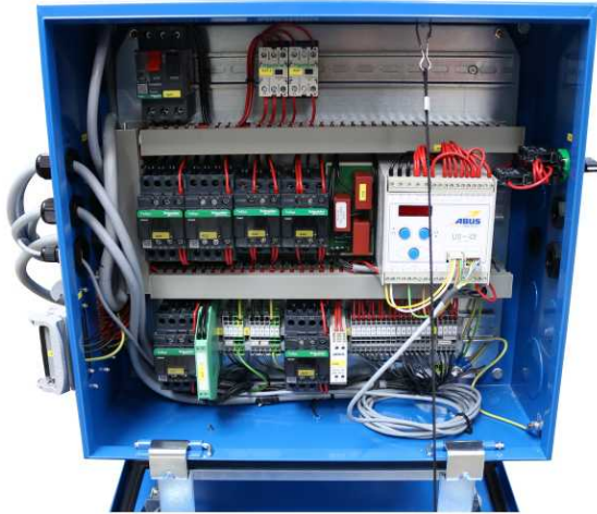
ABUS electrics 3 with contactor control
